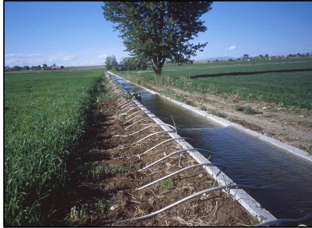
Lined Ditch with Siphon Tubes
